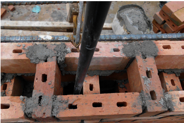
Electrical conduit passing through vertical cavities.
