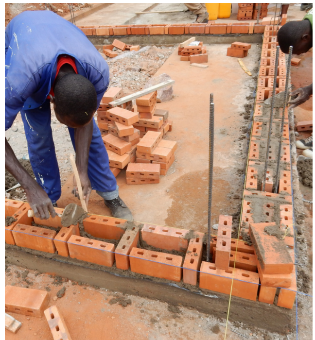
Masons laying the first row of RLB bricks
