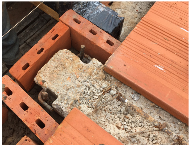
Detail of the Maxspan beam connection to the tie beam underneath.
