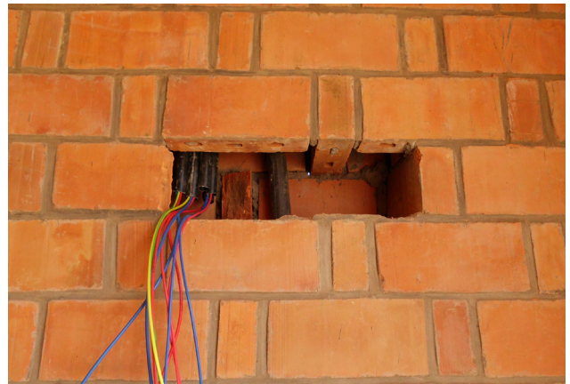
Electrical conduit and wires embedded in the a RLB wall.
