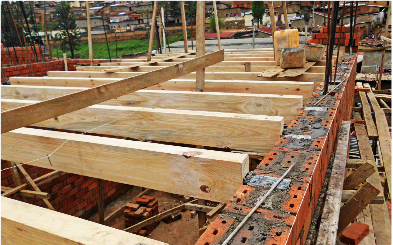
Example of a timber beams floor being installed on a RLB masonry wall system.
