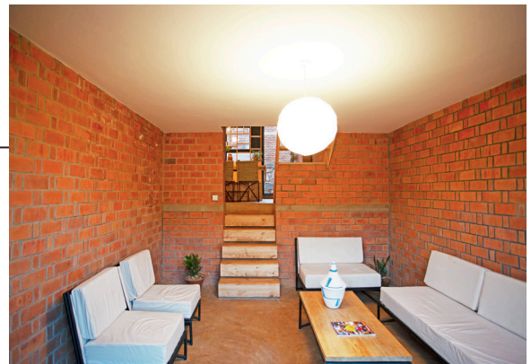
The Maxspan slab bottom surface plastered and painted.
