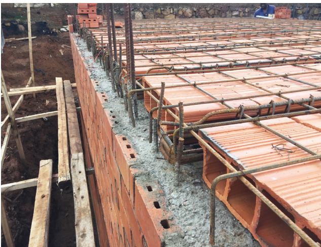
Detail view of the connection between the steel reinforcements and the tie beam underneath.
