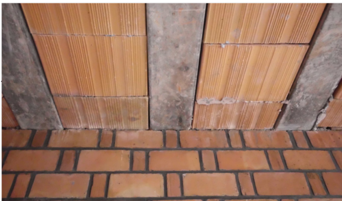
The Maxspan slab bottom surface without finishing.
