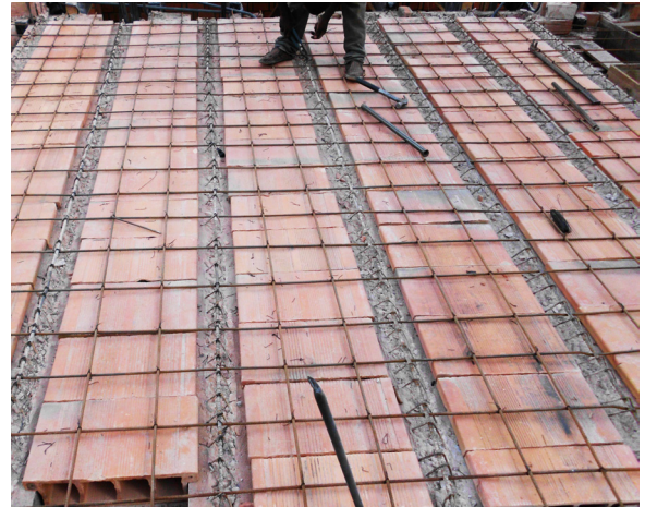
Top screed reinforcement mesh anchored to the pre-cast beams.
