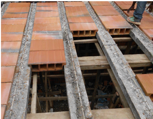
Maxspan blocks placed within the pre-cast beams.
