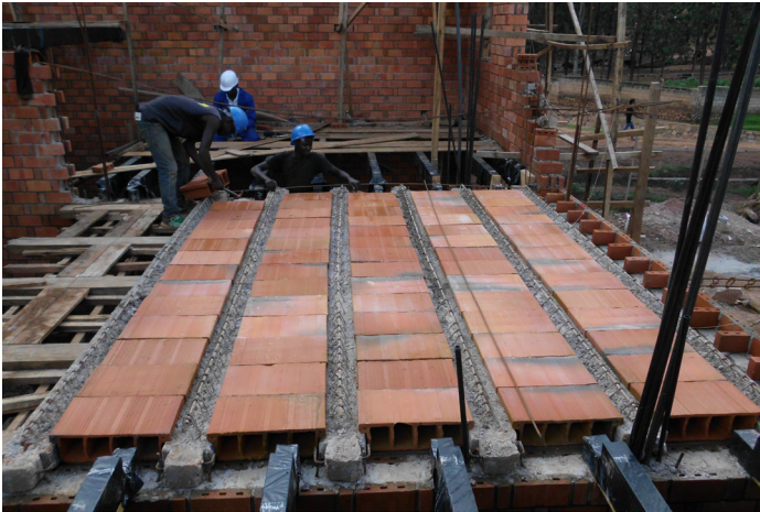
Maxspan blocks playing within the pre-cast beams.
