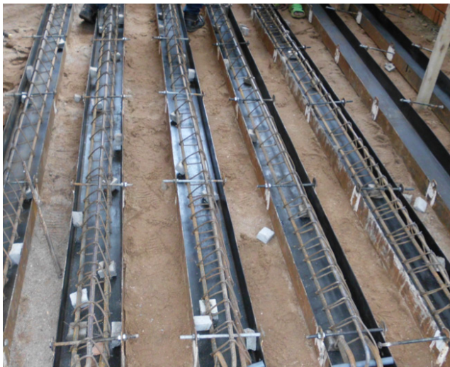
Maxspan formworks ready for concrete to be poured.
