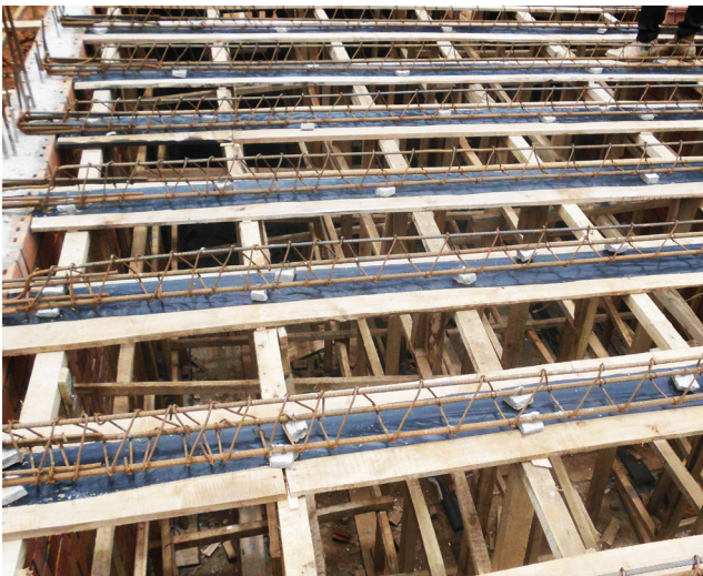
In-situ reinforcement positioned on the timber form-works.
