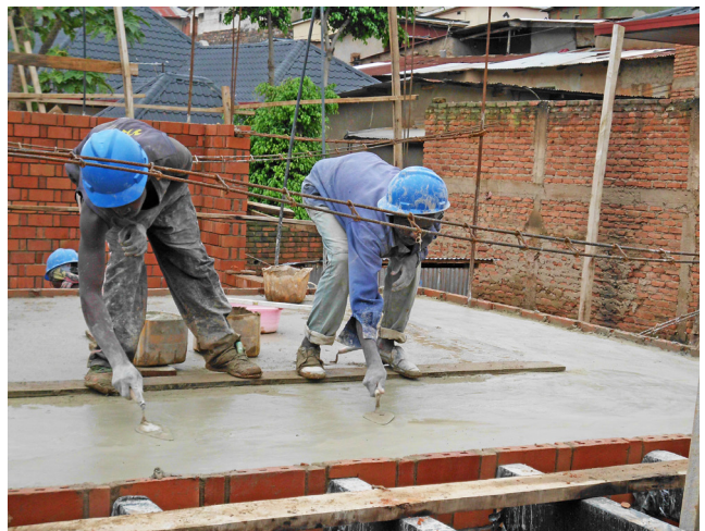
Finishing works after the final cement concrete layer is cast.
